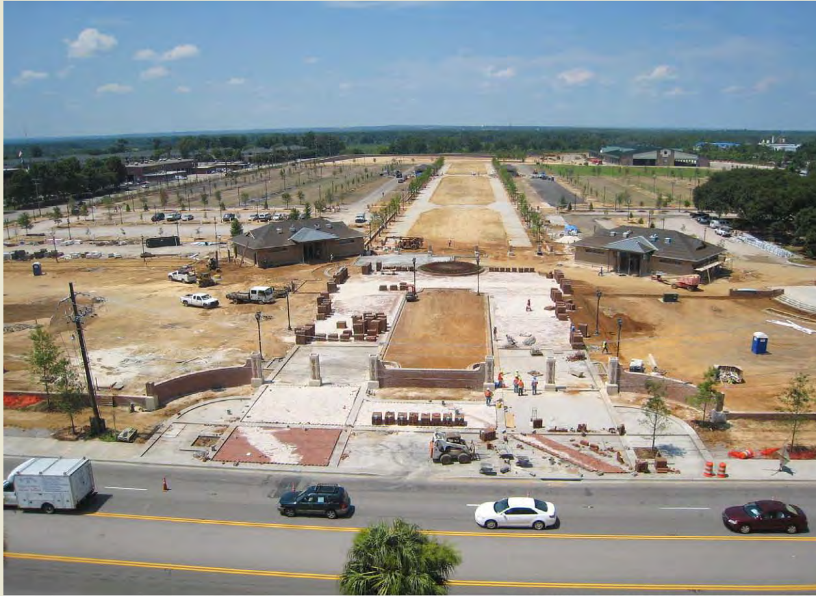
View of Gamecock Park under construction.
